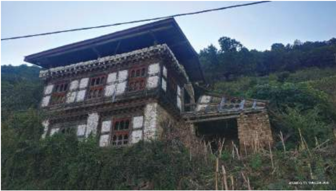
Figure 41: An abandoned house caused by Gungtong in the BC 9
