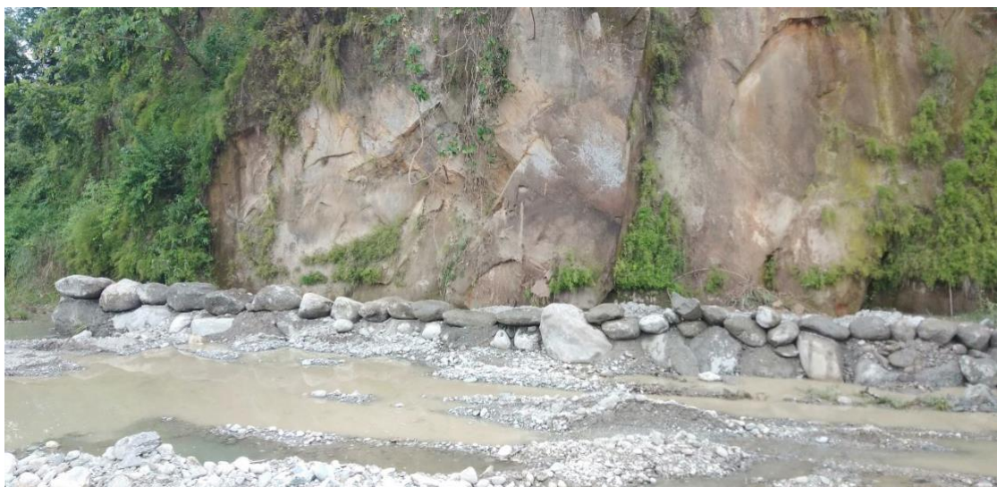
Figure 6 River bank protection
