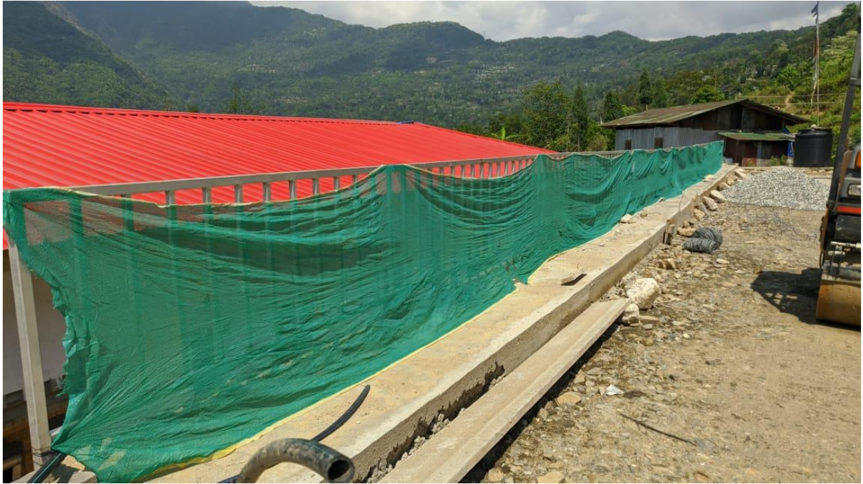
Construction site well covered to avoid disturbance to the Primary School
