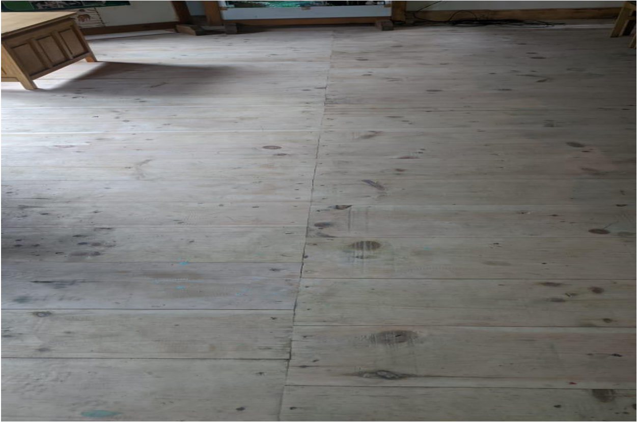
Well done flooring work by local contractor
