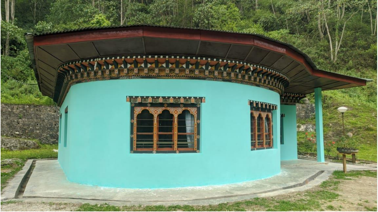
Renovation work is well executed at Rimchu Range office
