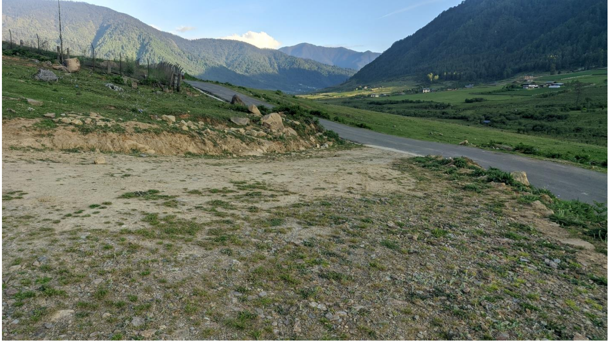
Parking space constructed by BC2 in Phobjikha Ramsar site
