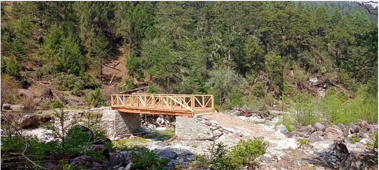
Bridge constructed by JKSNR with well-maintained surrounding
