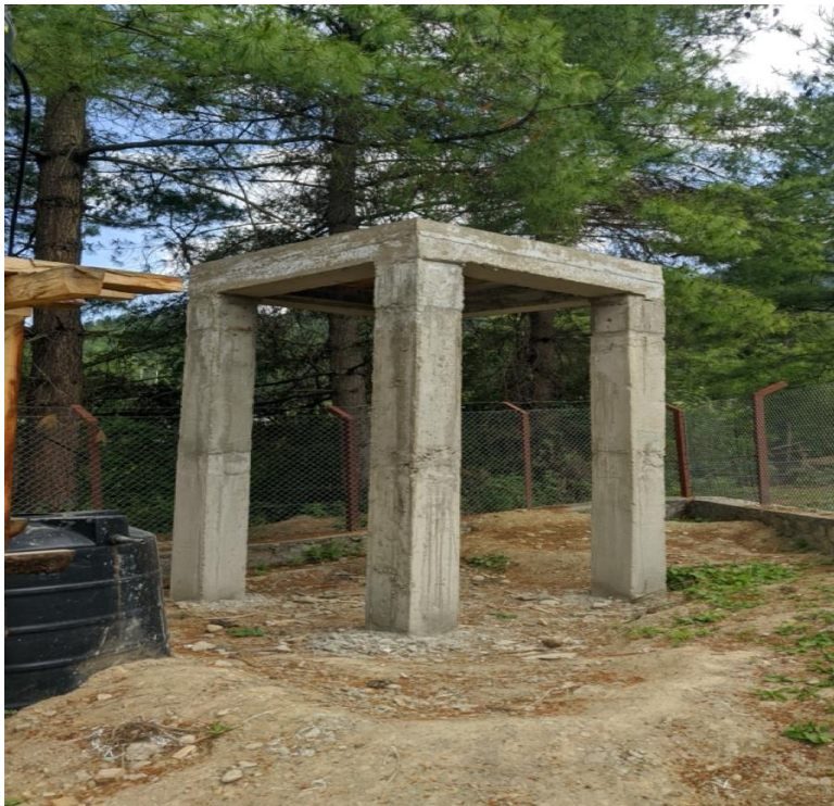
Water storage stand constructed by BC1 under Tsento Range Office in Paro
