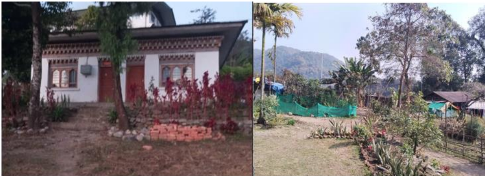
Figure 4- Present structure of Nganglam Range Office and the site status
