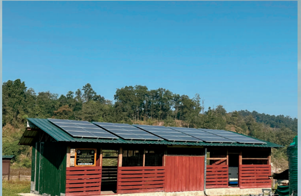
Photo 18: Solar Panel installed at Phibsoo Outpost Forest camp
