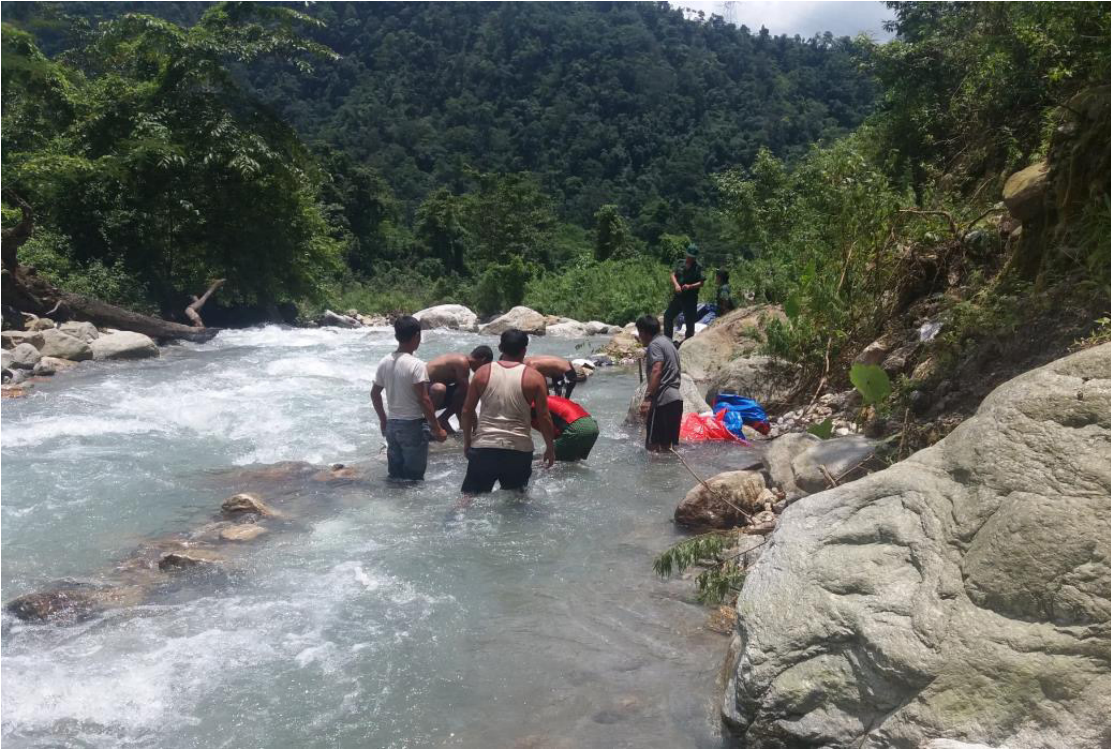
Figure 6. Illegal river training works executed by the local communities.
