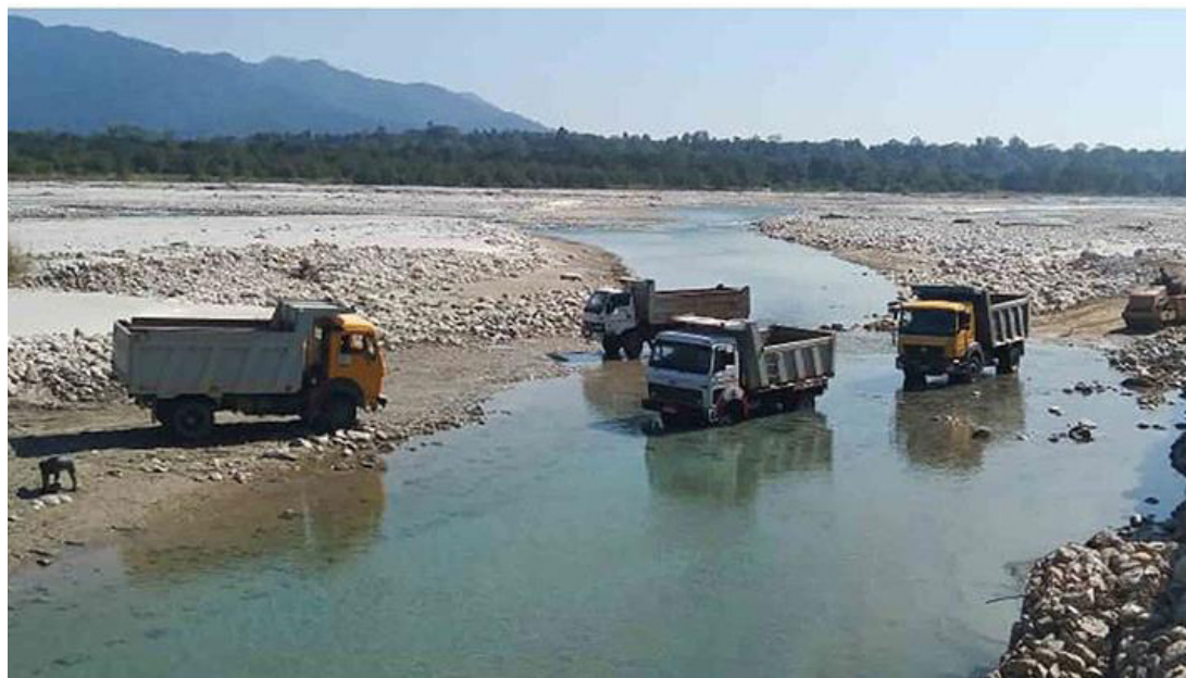
Figure 5. Dredging evidence by the side of Mahseer water.
