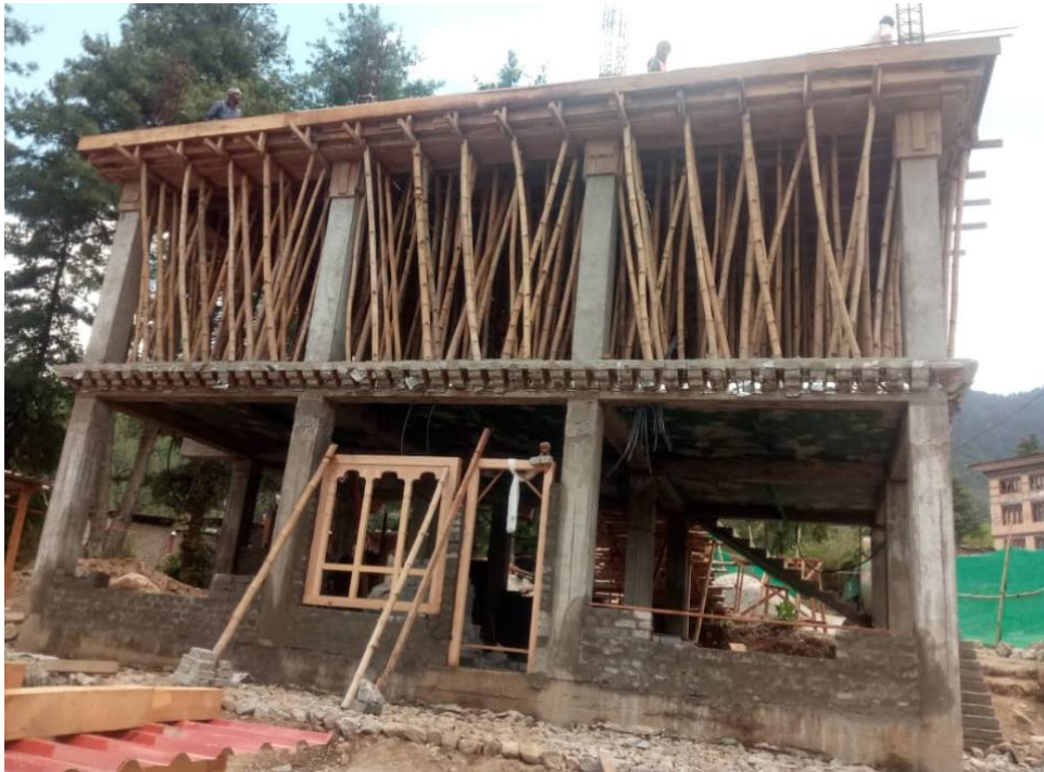
Figure 3: Ongoing construction progress at site
